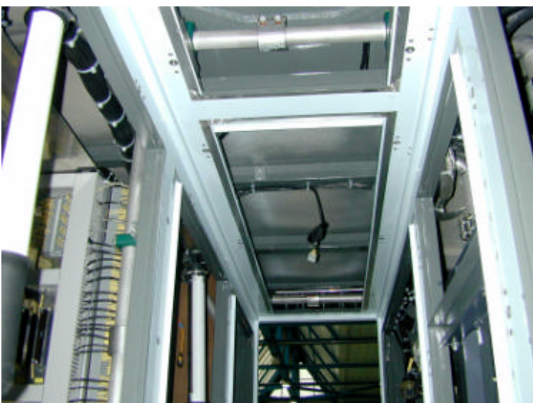
Oil conditioning for frequency converter water/ Glycole (Antifogen N, 60°C) STRAUB-METAL-GRIP 60.3 mm, EPDM
